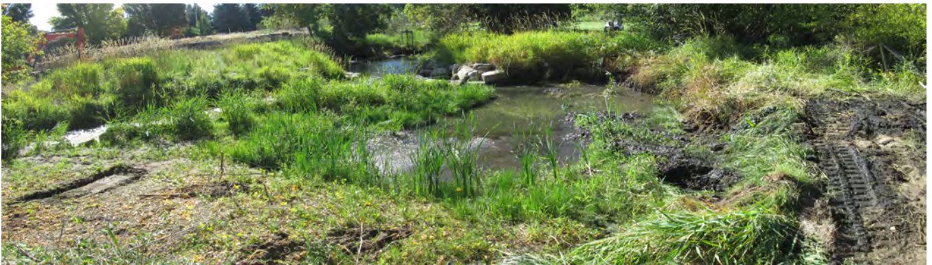
Photo 2. South view of on-going removal of the rock wall around the pond for backfilling. Photo taken September 15, 2023.
