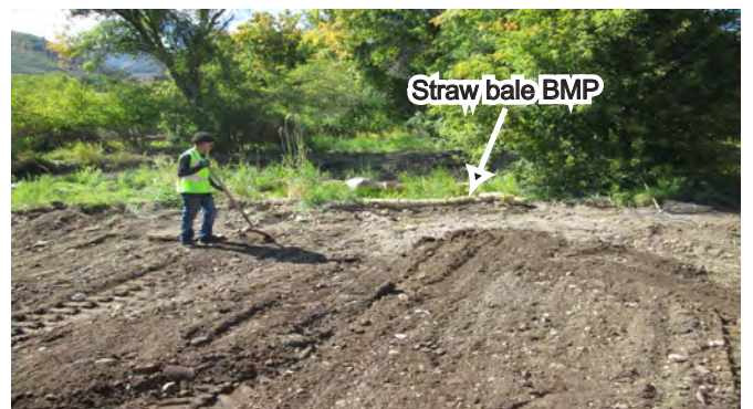
Photo 6b. Southwest view of straw bale BMP placed in fill removal area to protect Snake Creek. Photo taken on September 15, 2023.
