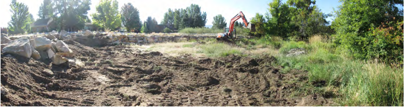
Photo 1. South view of fill removal in progress. Photo taken September 15, 2023.
