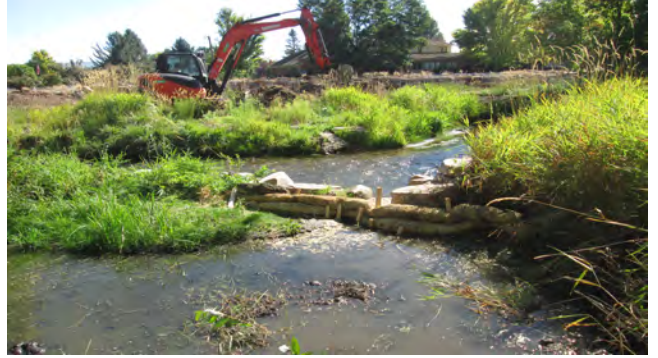
Photo 4b. South view of straw bale BMP to protect Snake Creek during back-fill of pond. Photo taken September 15, 2023.
