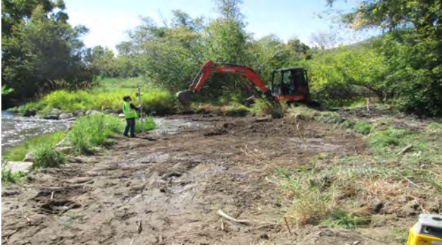
Photo 4a. South view of pond backfill being leveled using a laser-level. Photo taken September 15, 2023.
