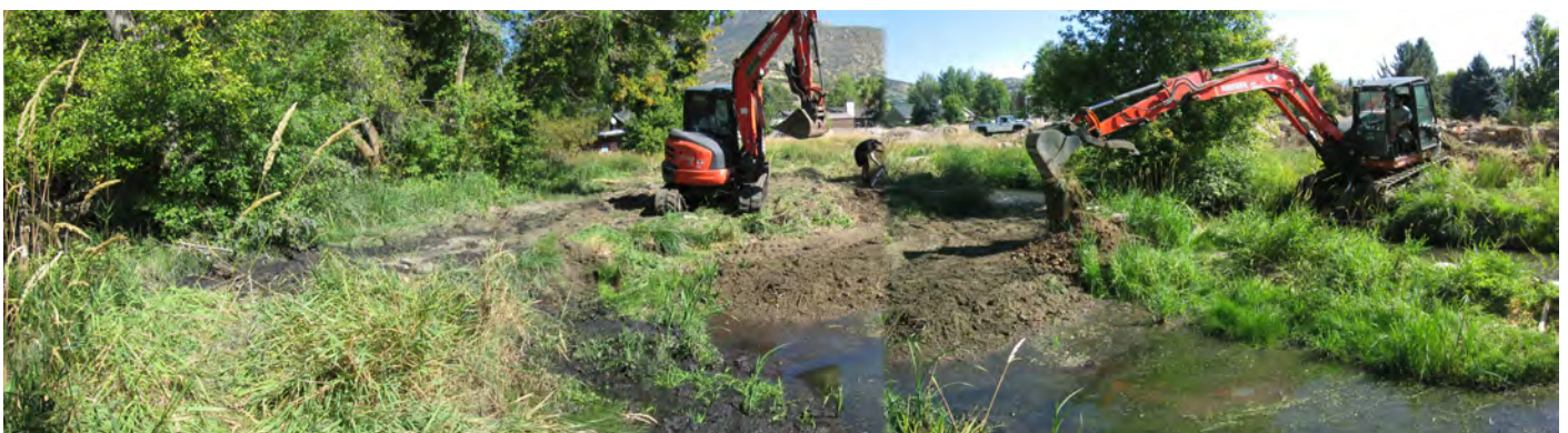
Photo 3. Northeast view of pond backfilling in progress. Photo taken September 15, 2023.
