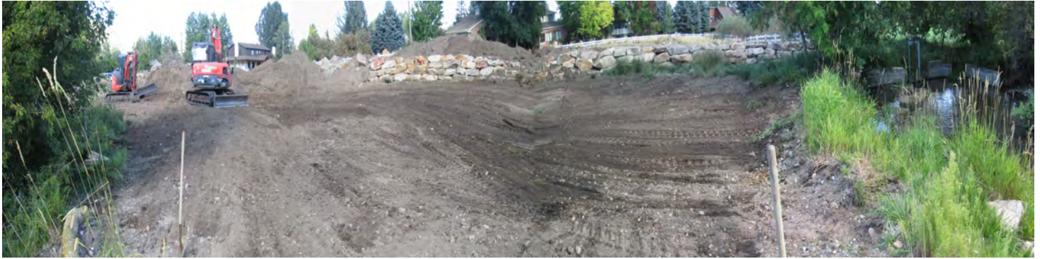
Photo 7. East view of completed fill removal in the fill removal area. Photo taken on September 15, 2023.
