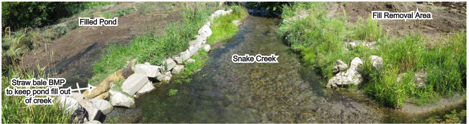
Photo 5. North view of backfilled pond (left), the straw bale BMP used to keep fill from entering Snake Creek (center), and fill removal area (right). Photo taken September 15, 2023.
