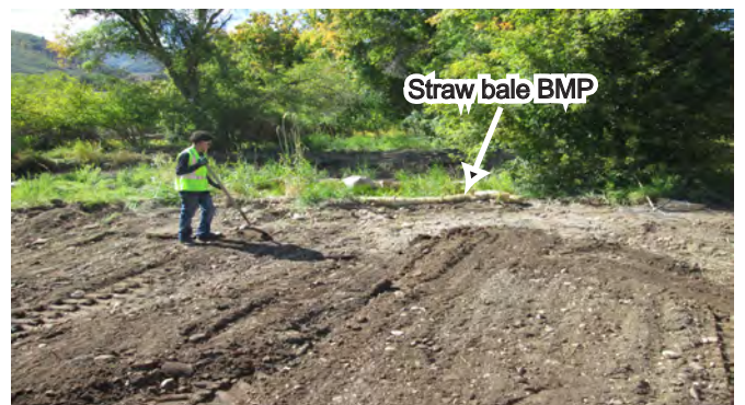
Photo 6b. Southwest view of straw bale BMP placed in fill removal area to protect Snake Creek. Photo taken on September 15, 2023.
